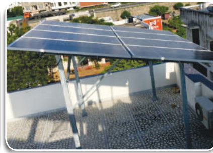
Rooftop Grid-connected SPV Power Plant at Residential building under Roof top Solar Power Generation Scheme 2019-20 of RREC
